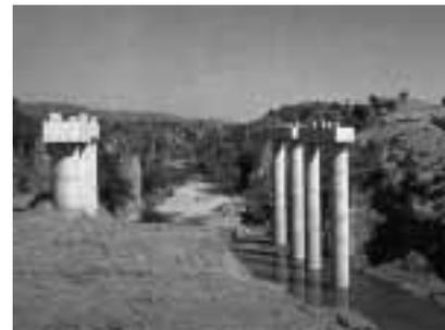
Fig 1: Fish unfriendly design. Piers located in midstream, abutments located too close to top of bank - eliminating riparian vegetation and causing pollution. Construction method pollutes river and destroys riparian vegetation.
